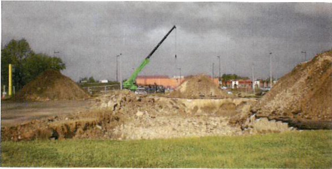
Fouille postes de distribution – 11-04-2012
